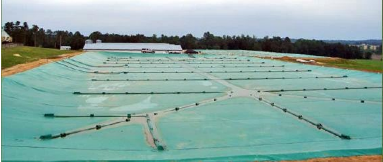
Photo of a covered manure lagoon. Source: US Environmental Protection Agency.
